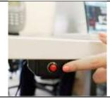
**Fixed Duress Button** – Press button to notify Security
